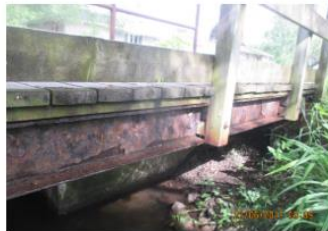
Photo 3: Exterior Steel Girder Supporting Walkway
