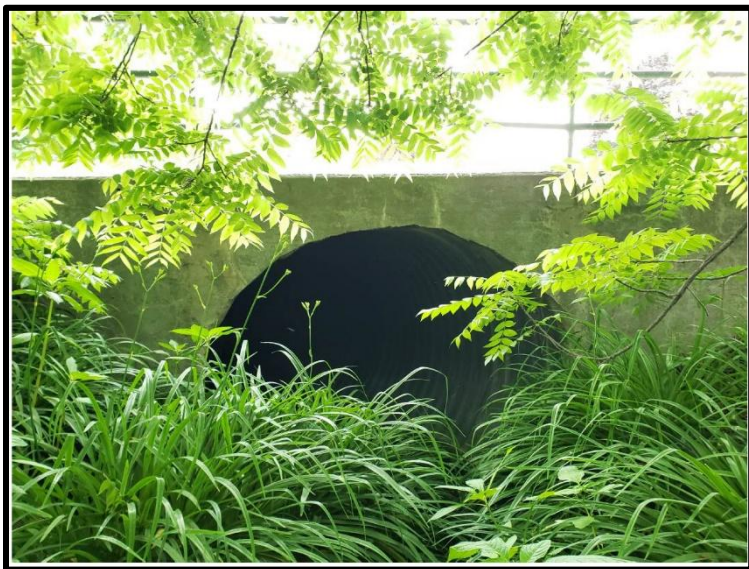
King Street Steel Culvert (BCI = 72 Good)
