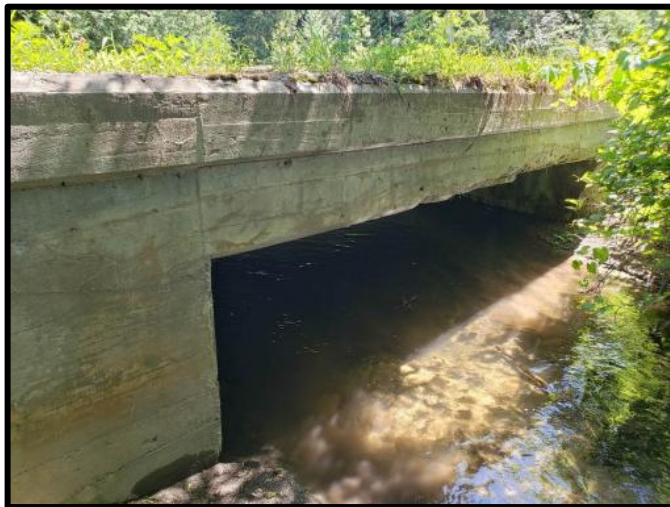
Ontario Street Bridge Culvert (BCI = 75 Good)
