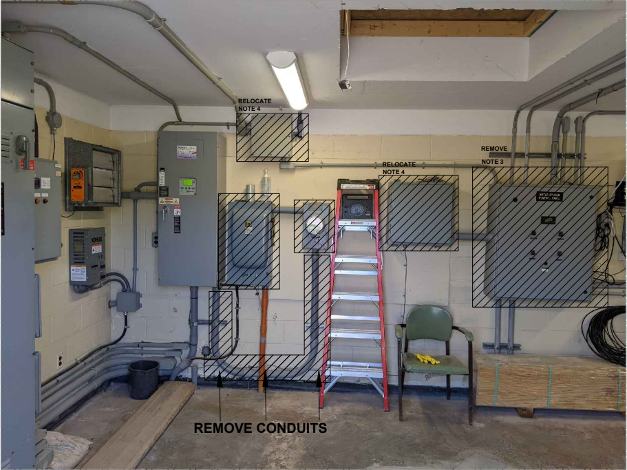
2 FRONT VIEW OF EXISTING DISCONNECT SWITCH AND POWER METER DEMOLITION
