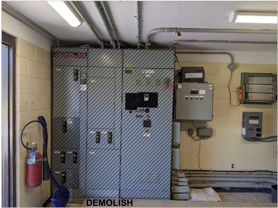
3 FRONT VIEW OF EXISTING MCC - DEMOLITION
