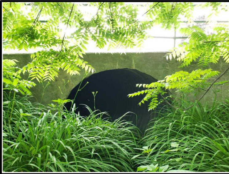
King Street Steel Culvert (BCI = 72 Good)
