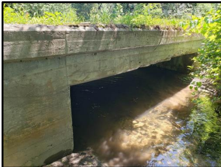
Dingman Road West Bridge (BCI = 48 Fair)
