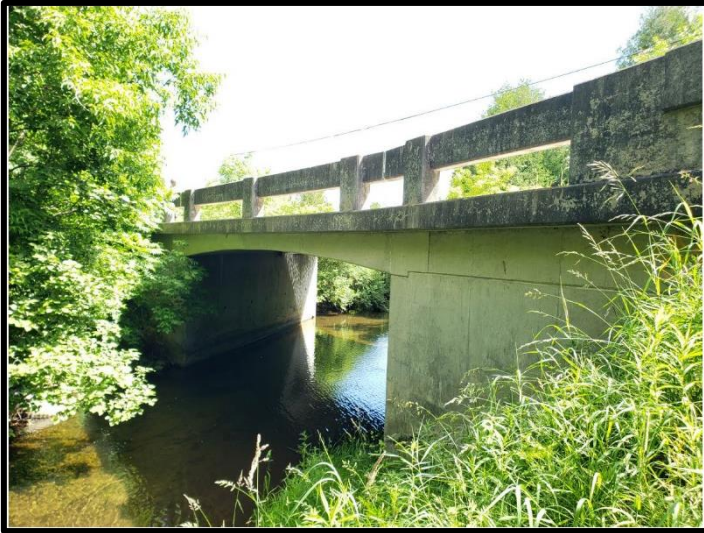
Campbell Road Bridge (BCI = 71 Good)
