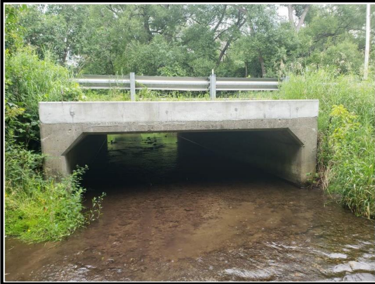
Ontario Street Bridge Culvert (BCI = 75 Good)
